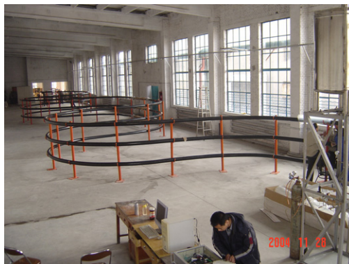
Figure 1. 75-m, 3 phase, 10.5 kV/1.5 kA HTS power cable installed at a substation.
